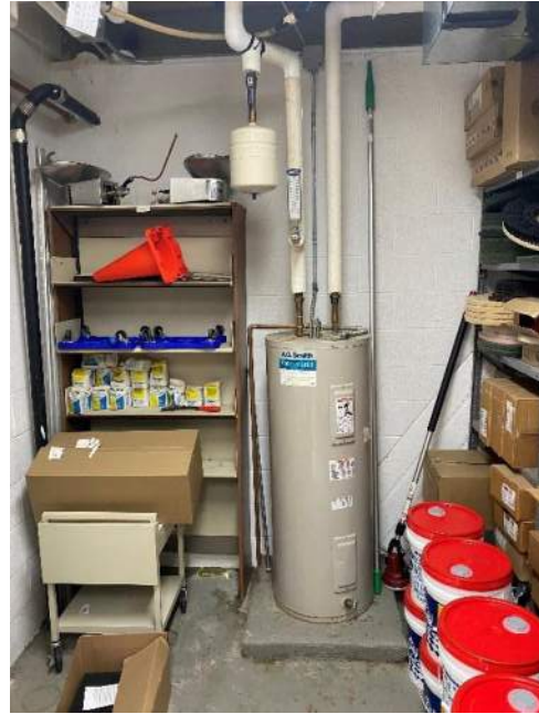
Electric Water Heater
