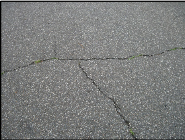
Unsealed pavement shrinkage cracks.
