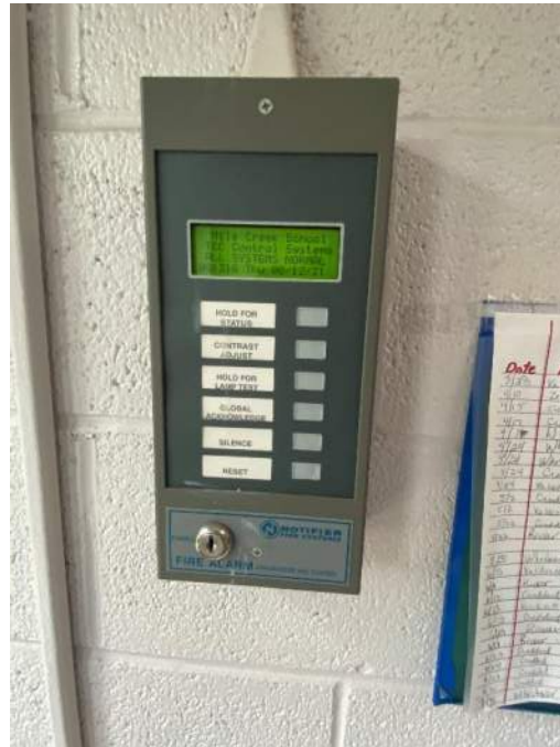
Remote Fire Alarm Annunciator
