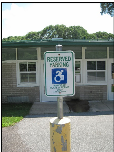
Existing accessible parking sign at Lot 1. Not compliant with CGS 14-253a subsection (h); CTBC Amd 1111.1
