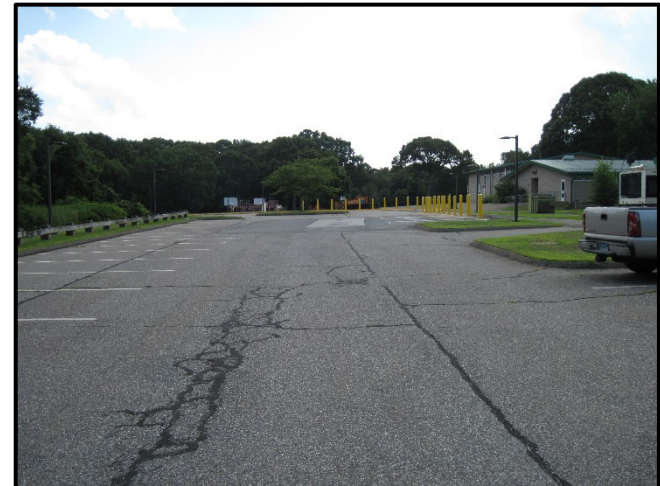
Lot 3 looking south. Sealed longitudinal cracks and fatigue cracks visible.
