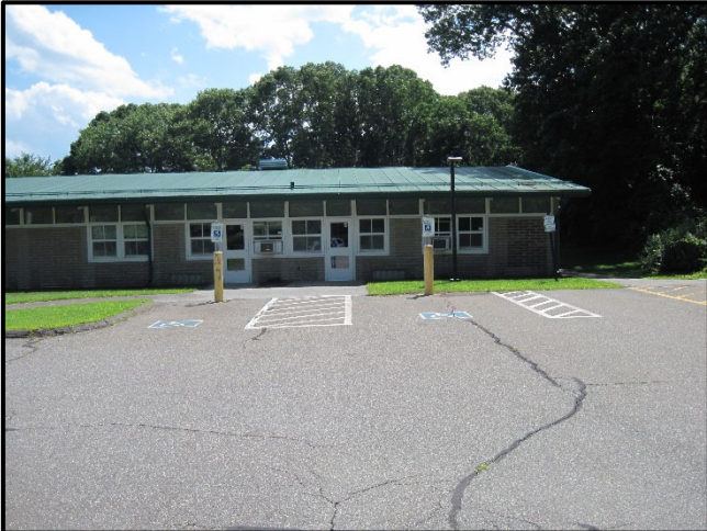
Existing accessible parking at Lot 1 (2 spaces). Right (west) access aisle not connected to "Accessible Route".
