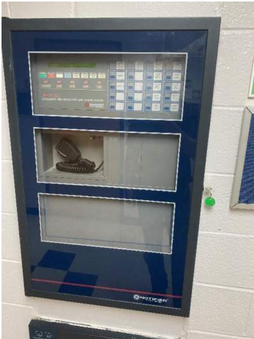
Fire Alarm Control Panel
