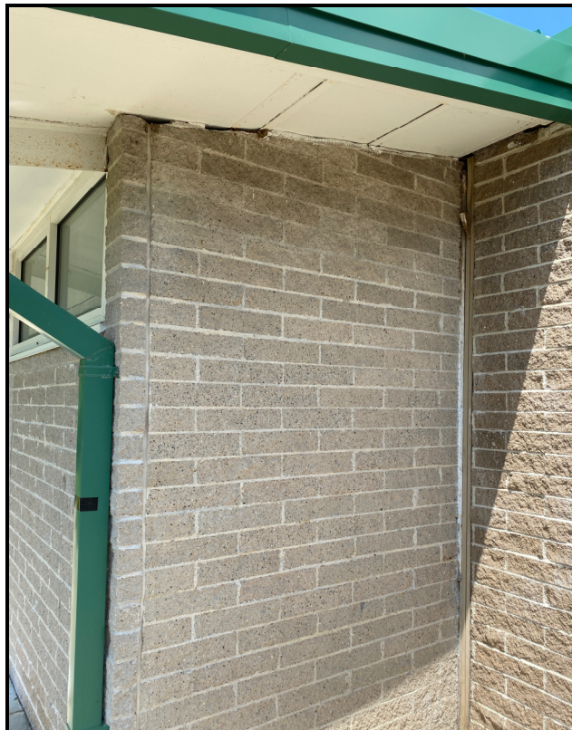
PHOTO 4: 7/23/2021 – Deteriorated caulking and rusted structural steel at soffit
