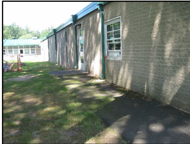
Looking north towards Door 15. Accessible means of egress must be compliant with IBC 1009.2, 1104, and ICC A117.1 Chapter 4, 402. Downspouts should be modified to eliminate discharge to walking surfaces.
