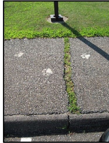
Shrinkage crack in bituminous walkway (at Lot 3).
