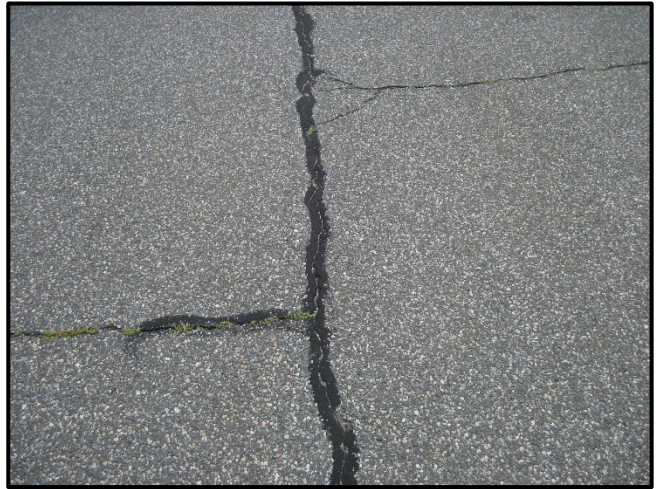
Typical failure of crack sealant. Additional crack propagation visible.
