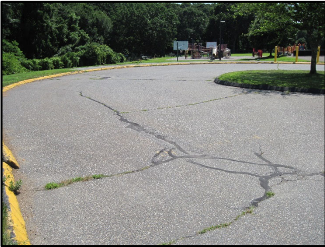
Sealed cracks and localized fatigue cracks visible.
