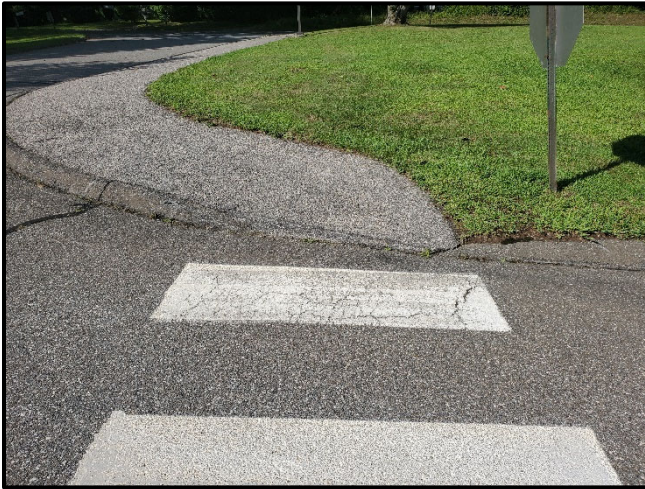
North curb ramp on east side of Drive 1 at Lot 2 crossing. Ramp is not in compliance with ICC A117.1, 406.
