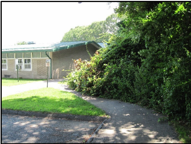
Bituminous sidewalk on west of side Lot 1. Vegetation should be cleared from walking areas.
