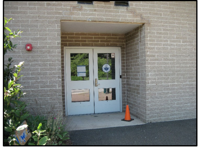
Typical accessible doorway, recessed, checked against ICC A 117.1 Chapter 4, 402 and 404.2.3.5.
