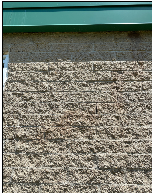
PHOTO 2: 7/23/2021 – Boiler Room – Mortar Crack
