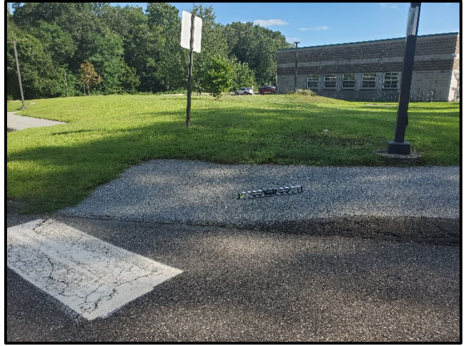
South curb ramp on east side of Drive 1 at Lot 2 crossing. Ramp is not in compliance with ICC A117.1, 406.
