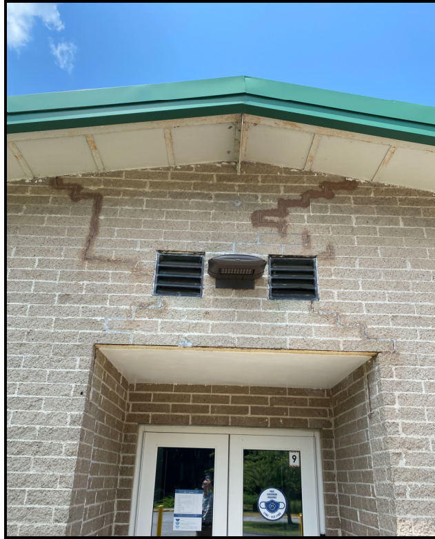
PHOTO 3: 7/23/2021 – Mortar Cracks at Vestibule 1121
