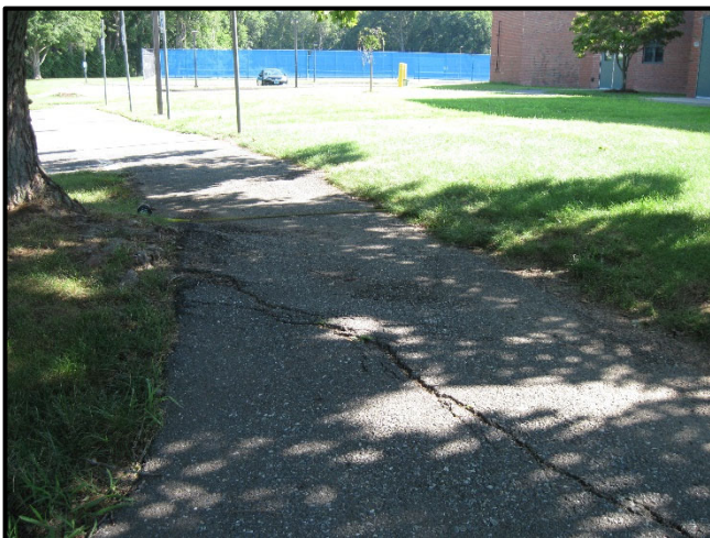
Walkway at front of school with heaving/root damage.
