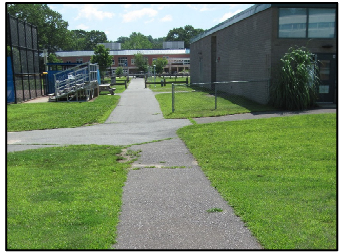
Bituminous site walkway, looking west from Door 7. Localized cracking and settlement visible.
