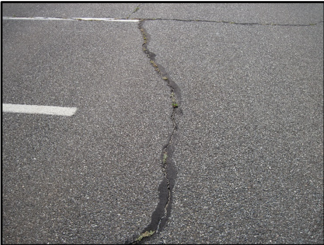
Typical failure of crack sealant.
