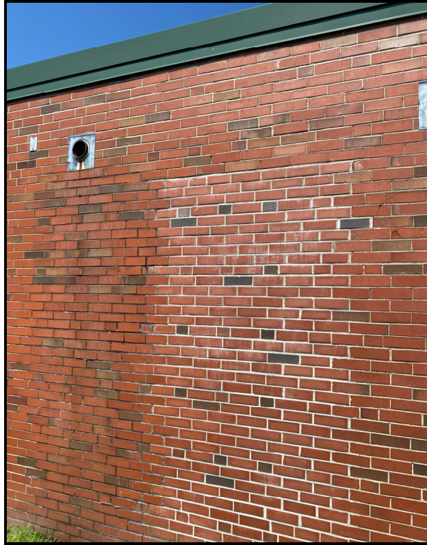
PHOTO 1: 7/23/2021 - Area D – East Wall - Cracked Brick and mortar joints requiring repointing.
