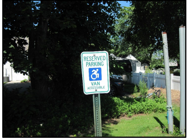
Existing accessible parking sign at Lot 1. Not compliant with CGS 14-253a subsection (h); CTBC Amd 1111.1.
