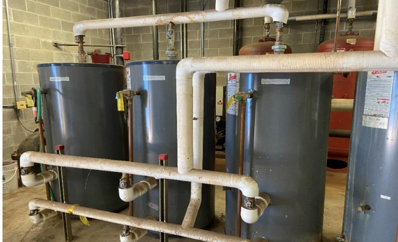
Domestic Hot Water Storage Tanks
