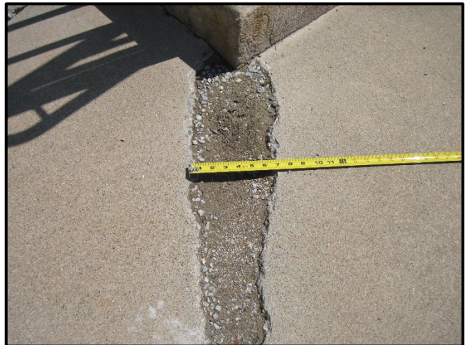
Pedestrian ramp 1, walking surface damage at top Landing.
