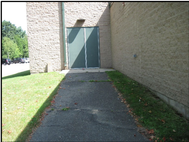
Accessible Route from cafeteria egress door. Cracks
