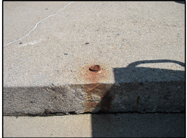
Stair 1, remnants of tubular post base in path of travel.
