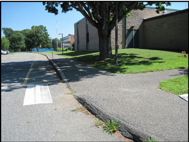
Curb ramp across from accessible parking in Lot 1 at crosswalk. Lacking 36-inch level landing.
