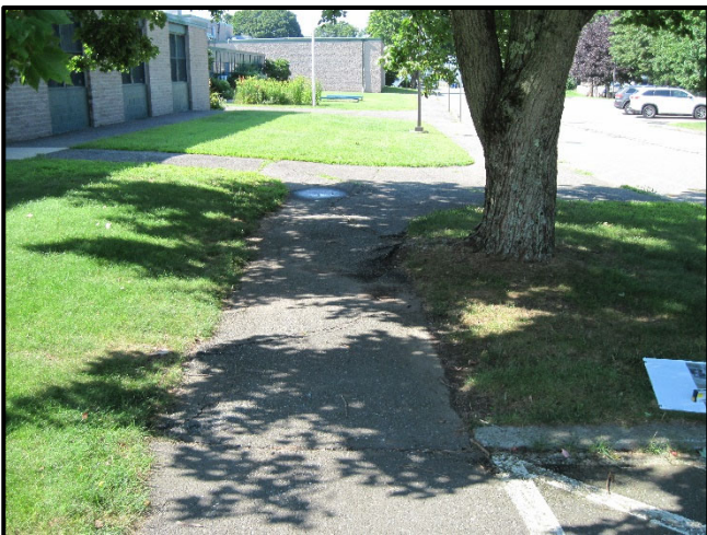
Walkway "Accessible Route" at Lot 3, looking south. Heaving and cracks from tree roots visible.
