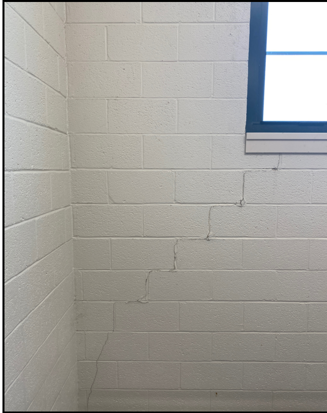
PHOTO 7: 7/23/2021 – Interior Stairwell – Settlement cracks
