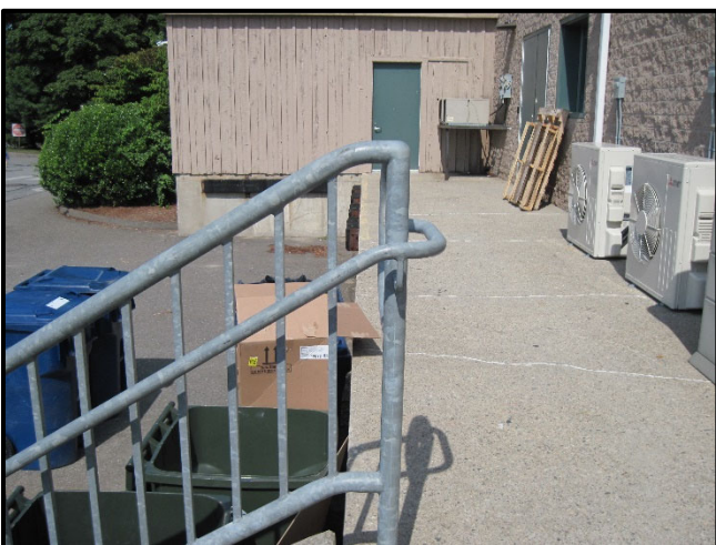
Stair 1, west rail, top rail extension.
