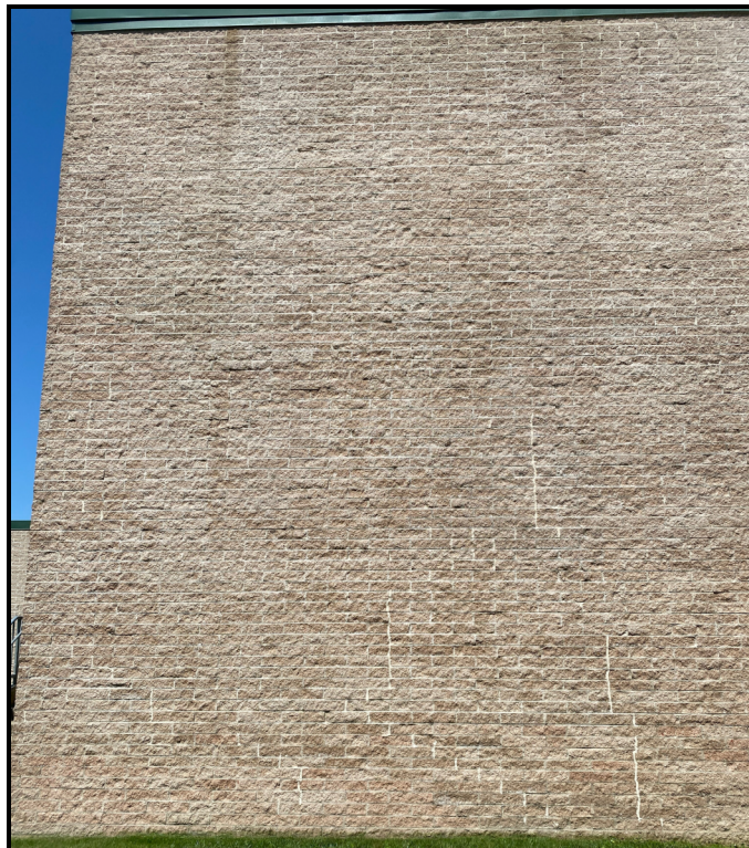
PHOTO 6: 7/23/2021 – North Elevation of Media Center – Cracked CMU caulked control joints
