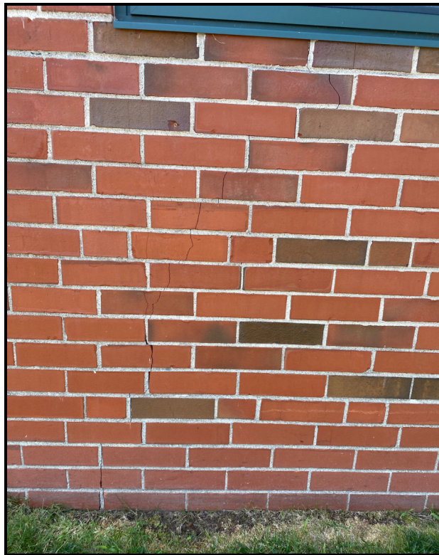
PHOTO 2: 7/23/2021 – Area D – East Wall - Cracked Brick
