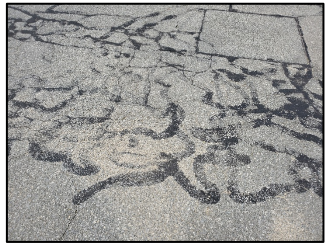
Localized area of block failure
