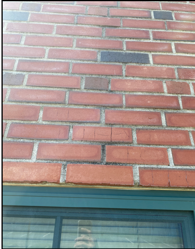
PHOTO 3: 7/23/2021 – South Elevation of Media Center – Cracked CMU and missing control joints
