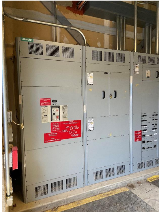
Main Switchboard at Electrical Room
