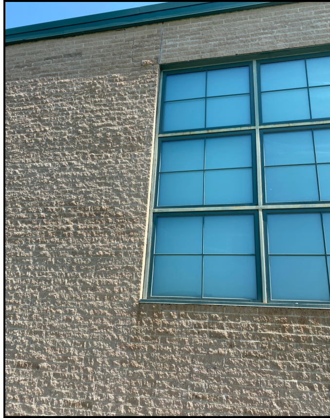
PHOTO 5: 7/23/2021 – South Elevation of Media Center – Cracked CMU and missing control joints
