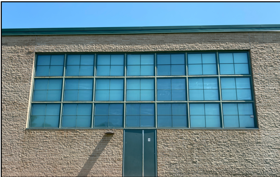
PHOTO 4: 7/23/2021 – South Elevation of Media Center – Cracked CMU and missing control joints
